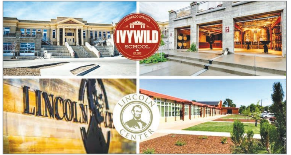
Ivywild and Lincoln Center are two adaptive reuse projects that are housing an array of unique local eateries. Both properties were formerly elementary schools.
