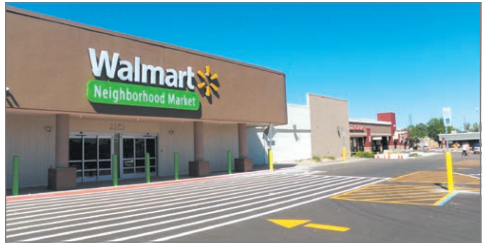
Renovation of Villa Monaco shopping center at South Monaco Parkway and Evans Avenue with anchor-tenant Walmart.
