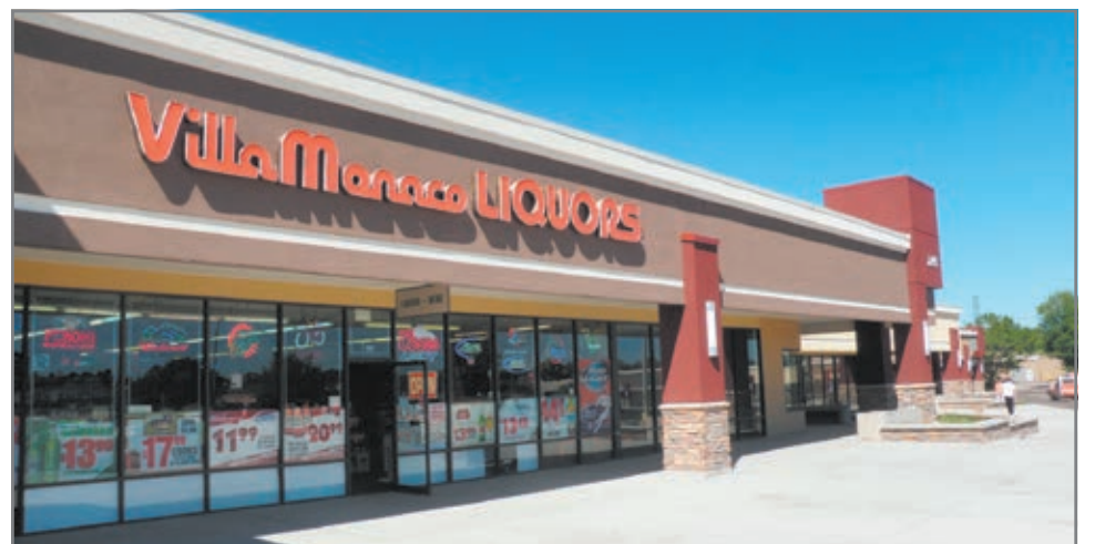
The Villa Monaco renovation continued throughout the center, providing a clean, updated look.
