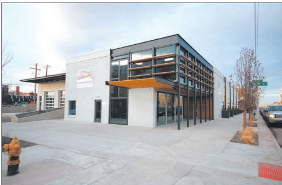
2601 Larimer is a mixed-used development with restaurant, retail and office space.
