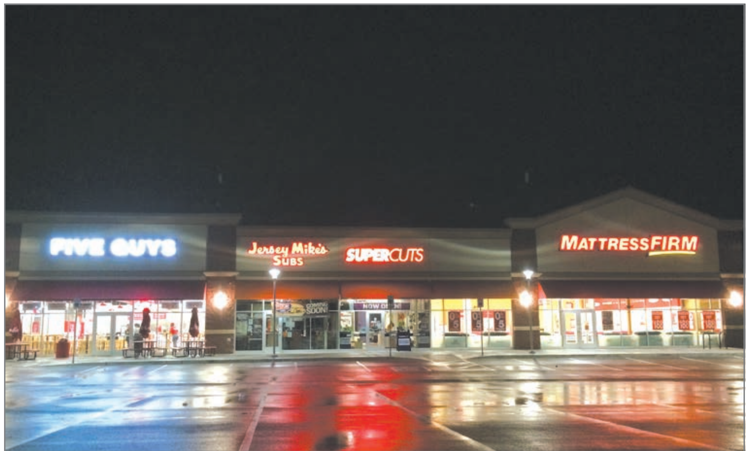
This strip mall was also completed as part of the project with Sprouts, which sold to an international company, represented by a California broker.
