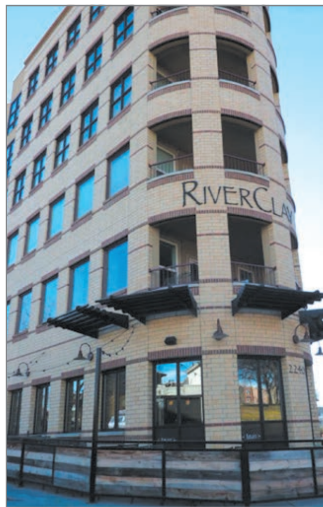
Many developments incorporate mixed-used elements with ground-floor retail space in apartment buildings, like at River Clay.
