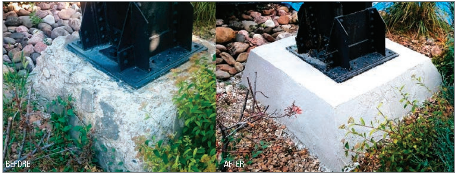
The applicability of concretelike polymer-based materials is widespread and can be beneficial when setting, securing or repairing areas around handrails, metal stair noses and footers.
