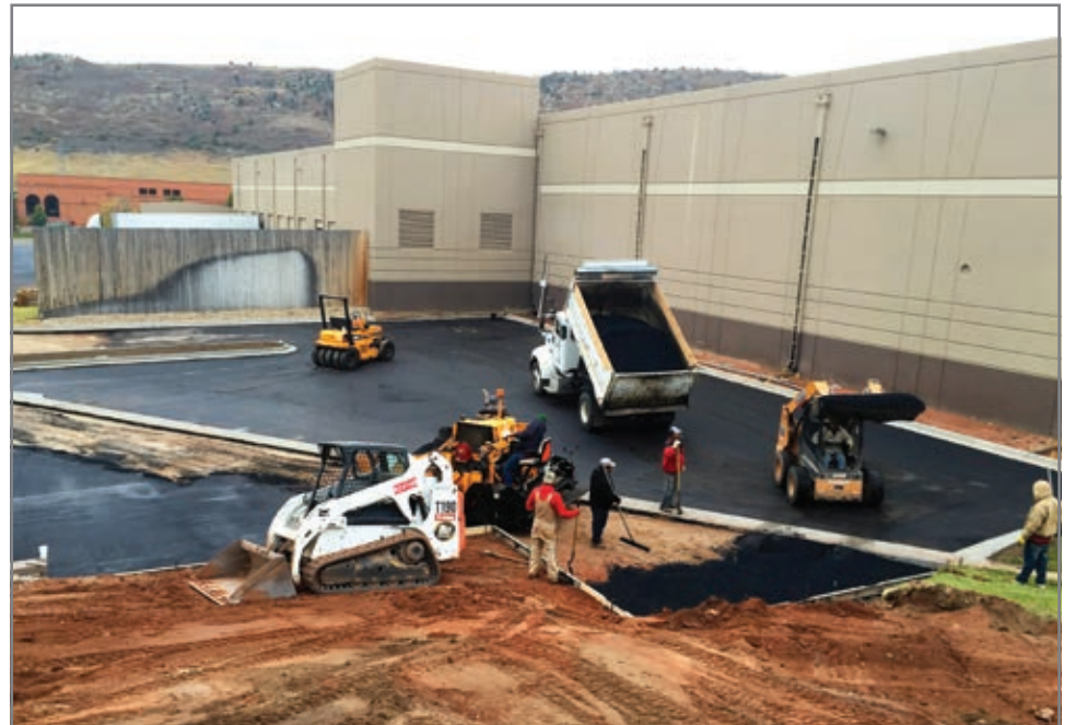
Economy Paving crews perform a full-depth replacement, which is the result of neglecting a parking lot for years and refusing to do maintenance practices to prolong the life of the concrete and asphalt.
