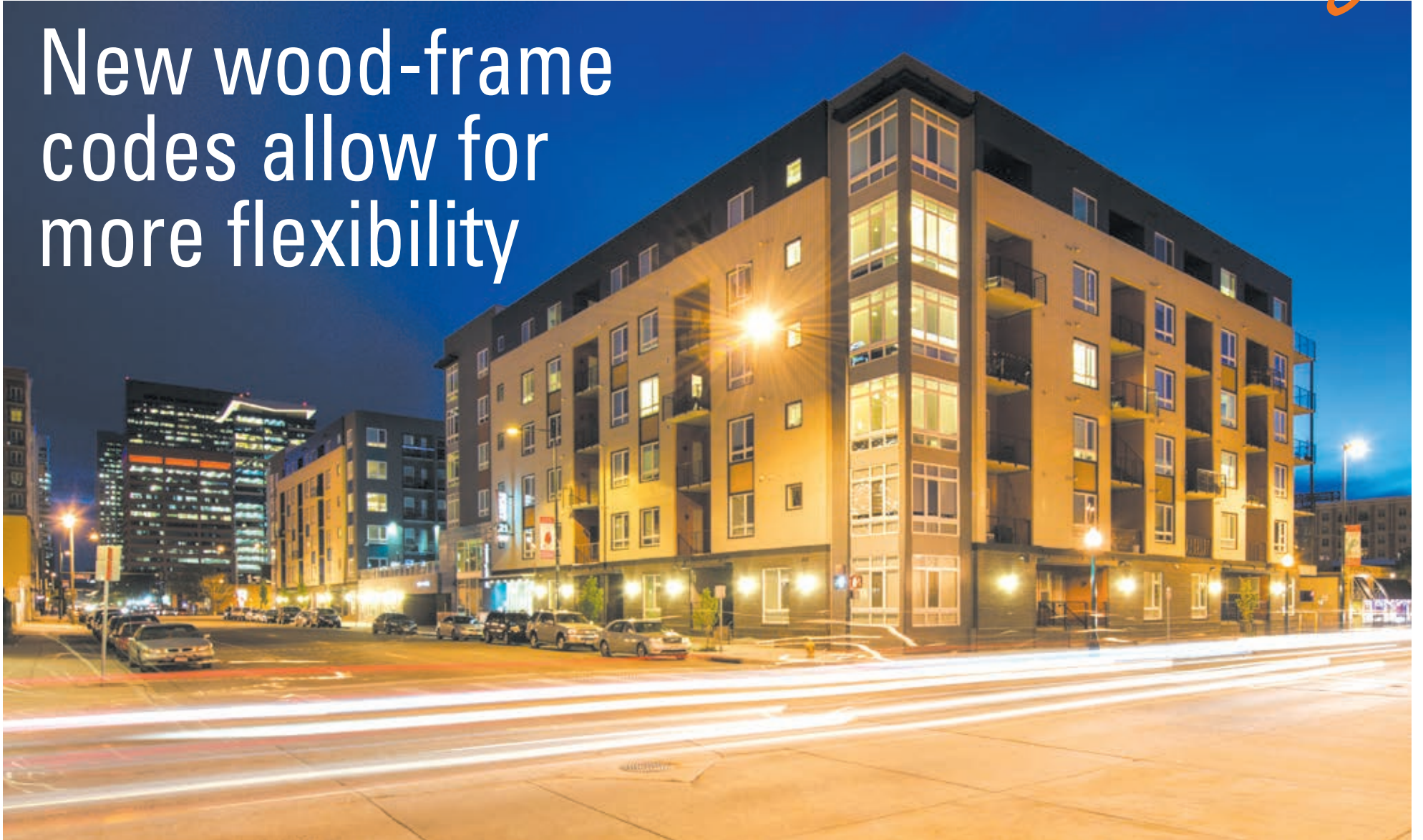
The 2015 International Building Code offers wood-frame construction the ability to design a podium building based on the overall building height. Podium buildings will no longer be restricted to only one level of podium structure below the podium deck. Photography © Brad Nicol
