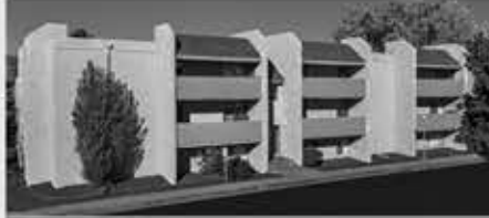
PINE CREEK VILLAGE | 312 UNITS
