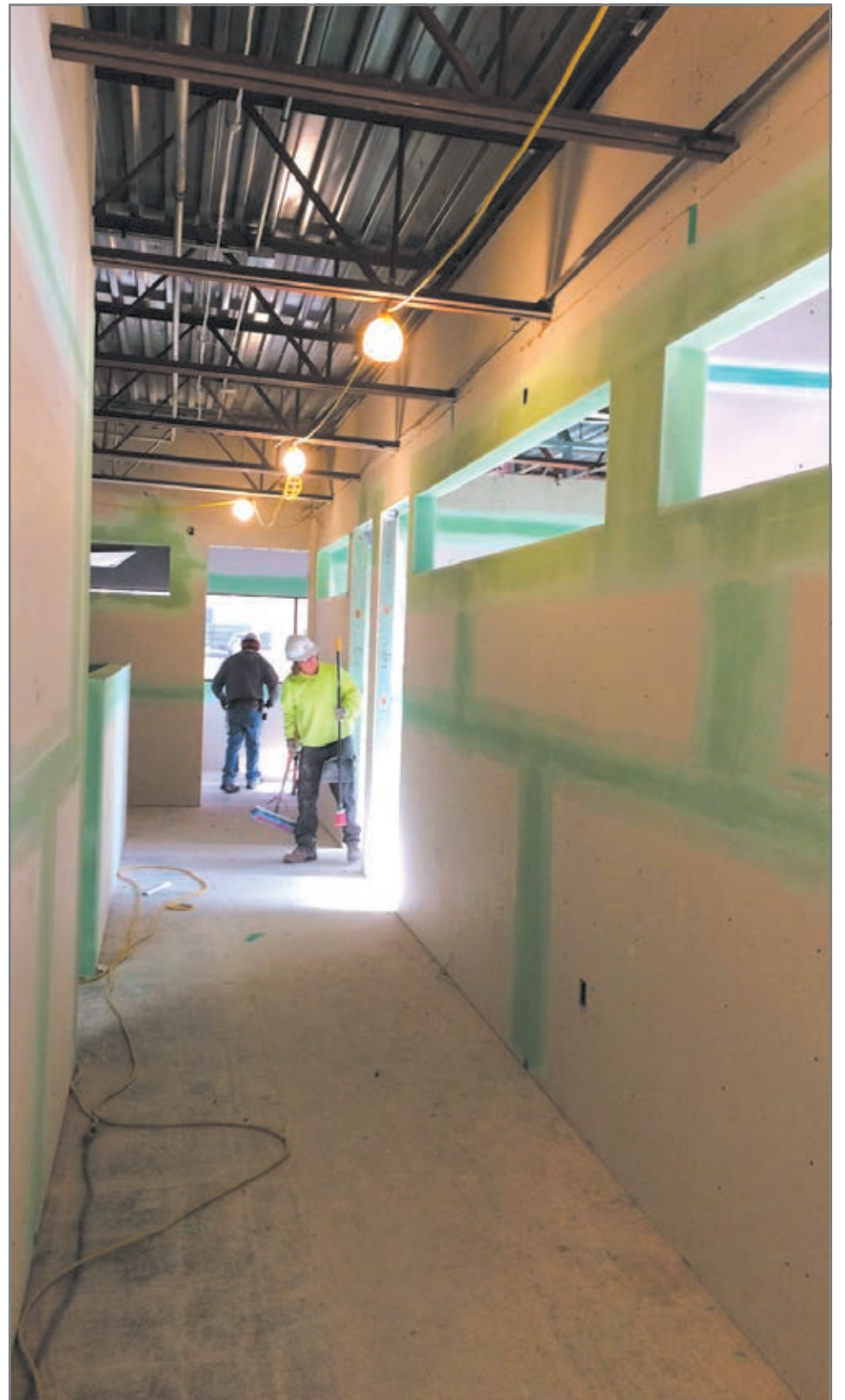
The removable drywall tape is used to be able to reconfigure spaces using the same materials.
