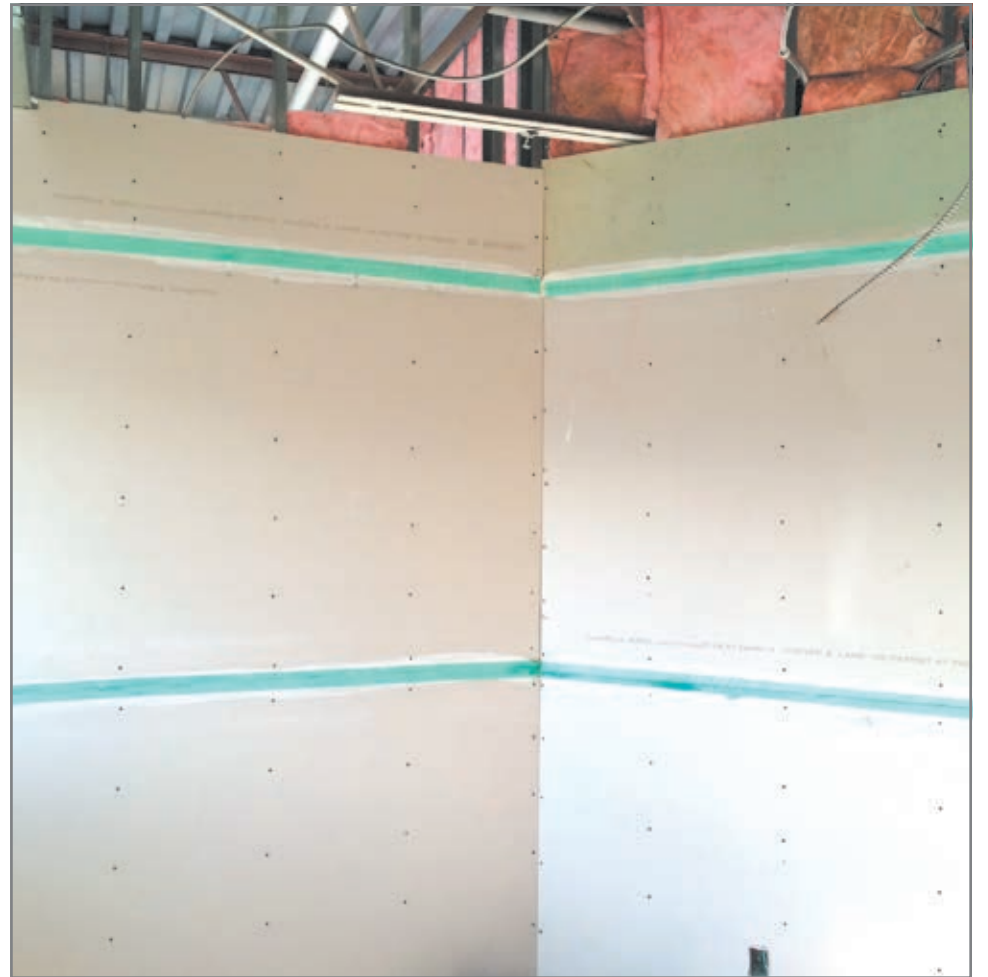
Green-Zip drywall tape adheres to drywall in the same fashion as regular tape but without the long drying time.
