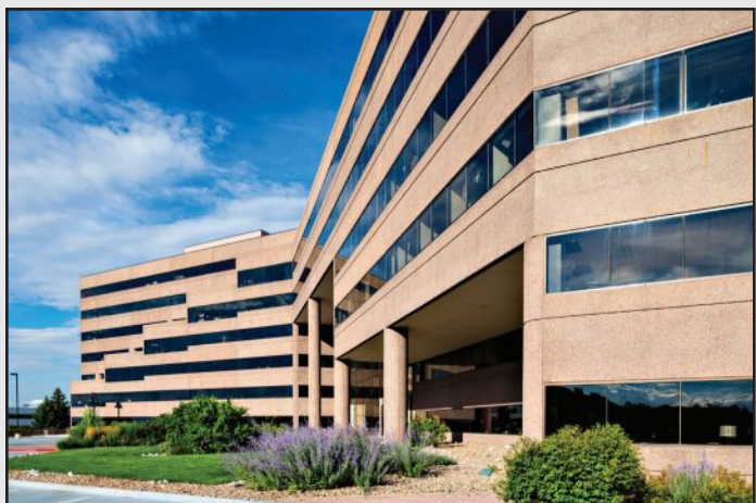
A seven-year, fixed-rate acquisition loan at 70 percent loan to value was arranged for the $63 million purchase of the Cascades office property in Centennial.
