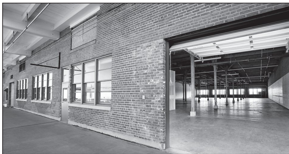
North Denver Industrial Park was built as the Denver Medical Depot, which began operating in 1942.
