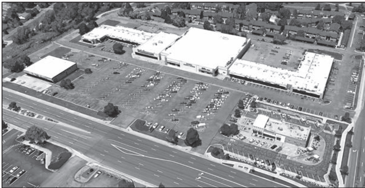
Shown is the Iloff Crossing Center
