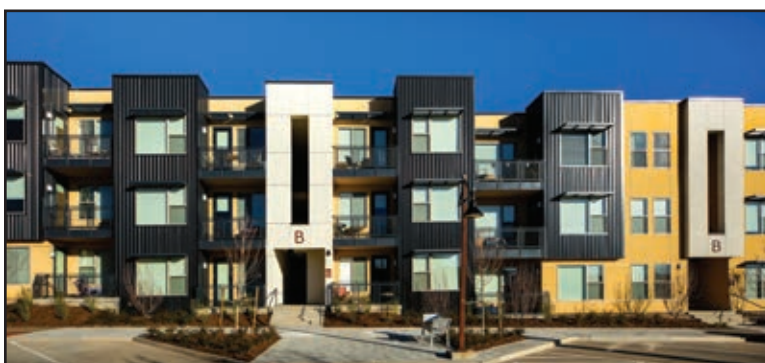
Confluence at Three Springs in Durango is the first new apartment community of its kind in 30 years.
