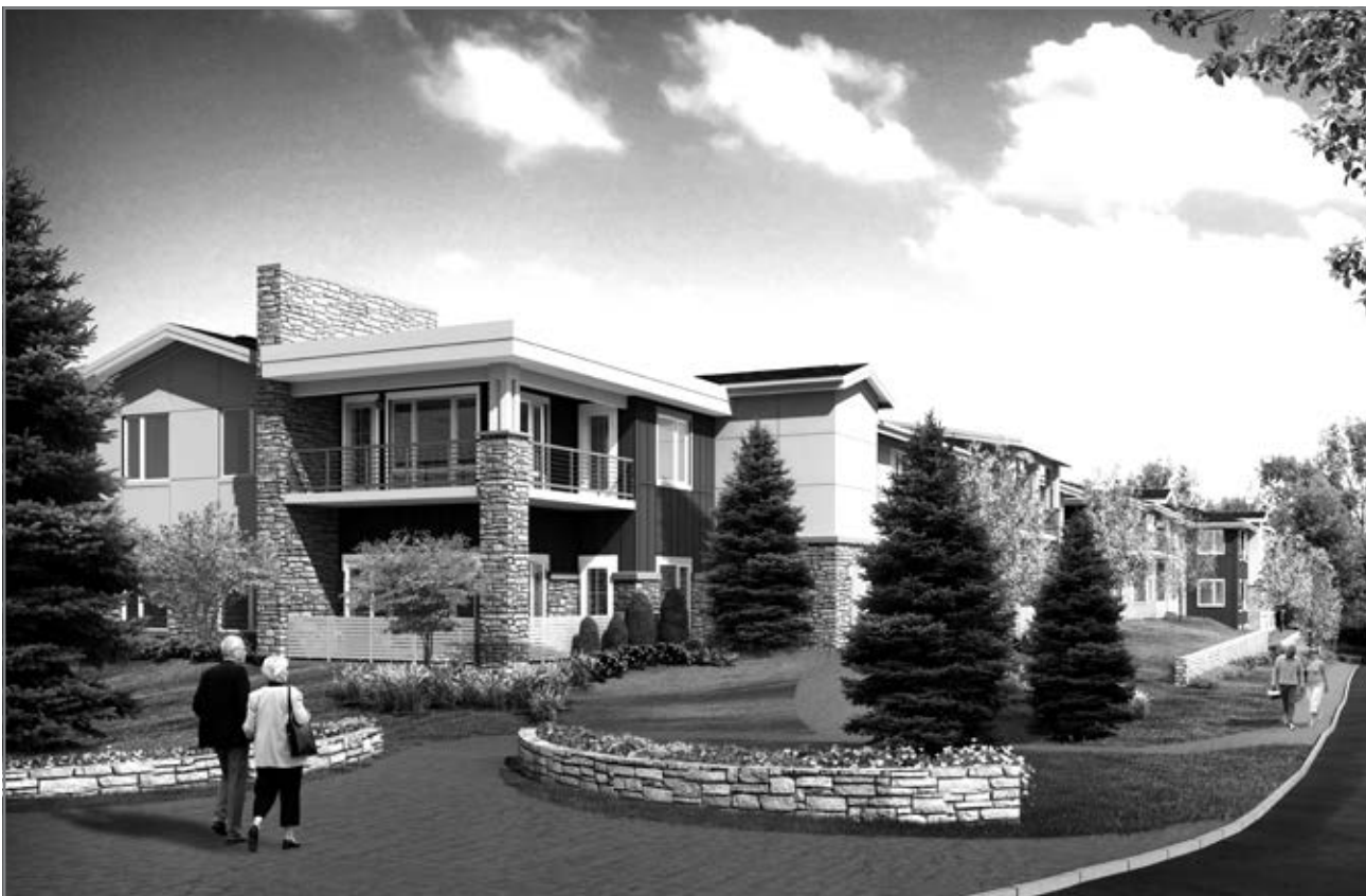
Legacy Village at Castle Pines is a 66-unit independent living, 79-unit assisted living and 31-unit memory care community. Site work began in August with an official groundbreaking ceremony in late September. The architect is Lantz-Boggio Architects and the general contractor is Shaw Construction. The property will be owned by Western States Lodging II LLC and is expected to open in October.
