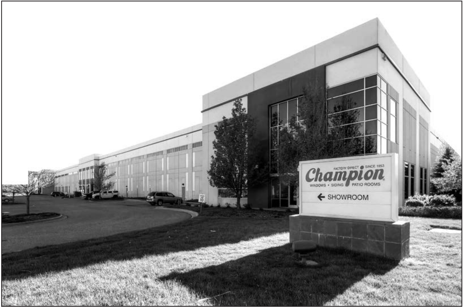
Champion Windows occupies about 116,000 square feet in the building at 10000 E. 45th St. in Denver.
