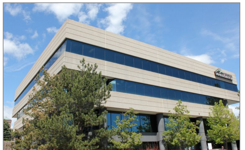
Rocky Mountain Gastroenterology leased 4,890 square feet in Lakewood.
