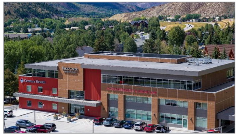
NexCore's Buck Creek Medical Plaza in Avon was one of five outpatient projects the firm completed in 2016.
