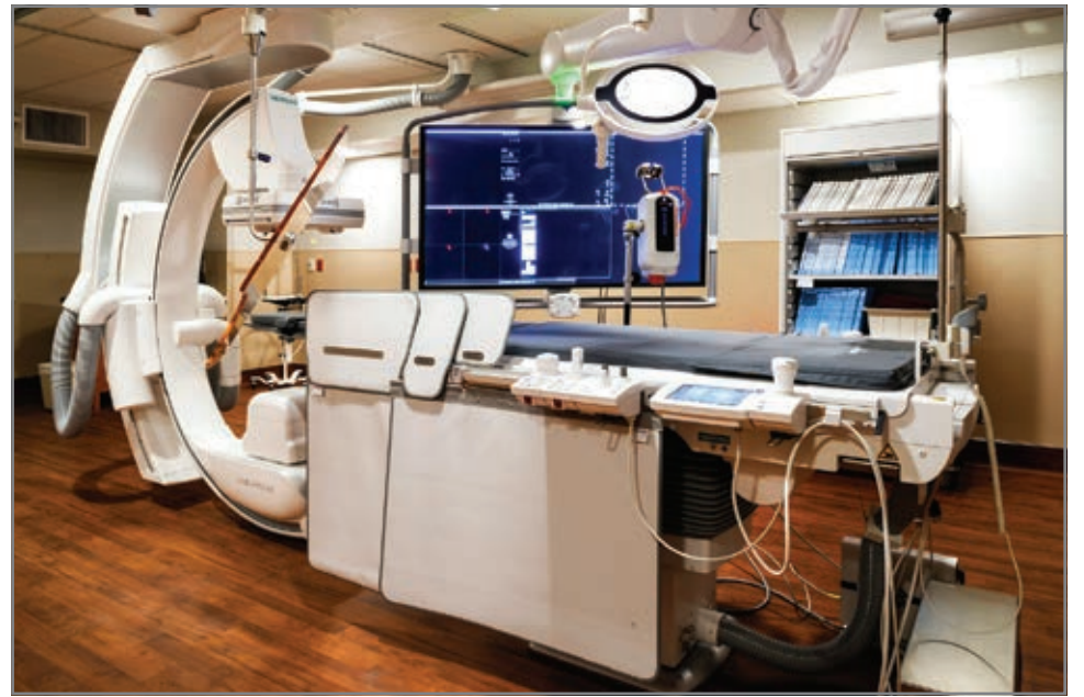
A look at the interventional radiology renovation completed by Catamount Constructors at Presbyterian St. Luke's.
