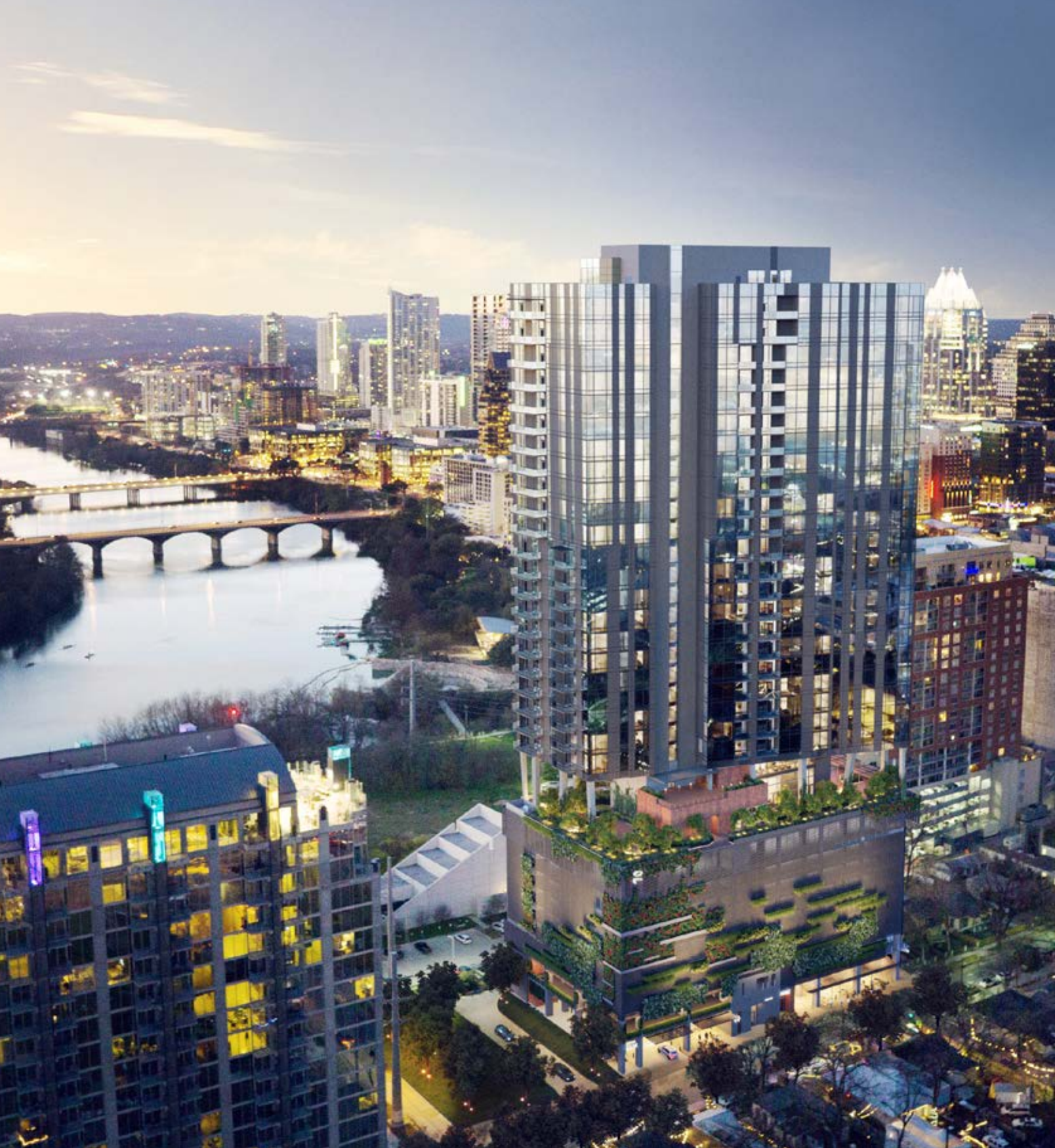
70 Rainey Street Condominium Highrise
