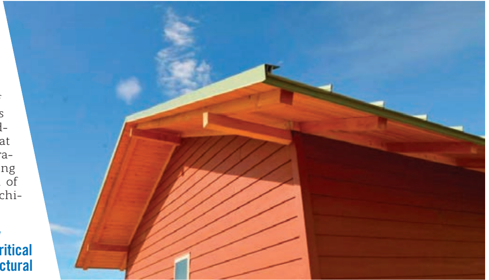
Pine Ridge Reservation’s Net Zero low-income housing integrates simple, elegant detailing to create dignified, higher-performance homes for comparable costs of doublewides and FEMA trailers.
