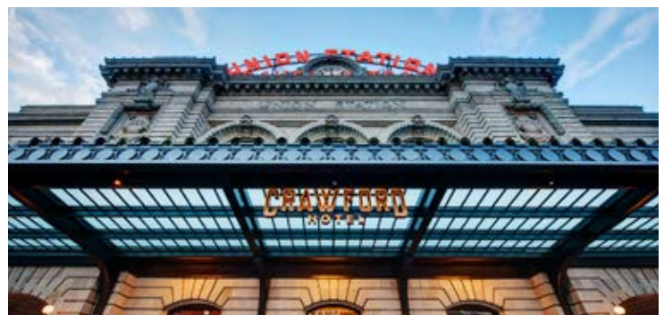
CRAWFORD HOTEL – Tryba Architects & Johnson Nathan Strohe
